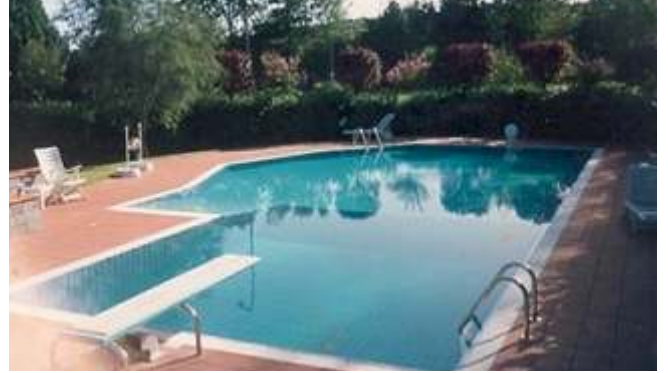
Overflow on a tile side
